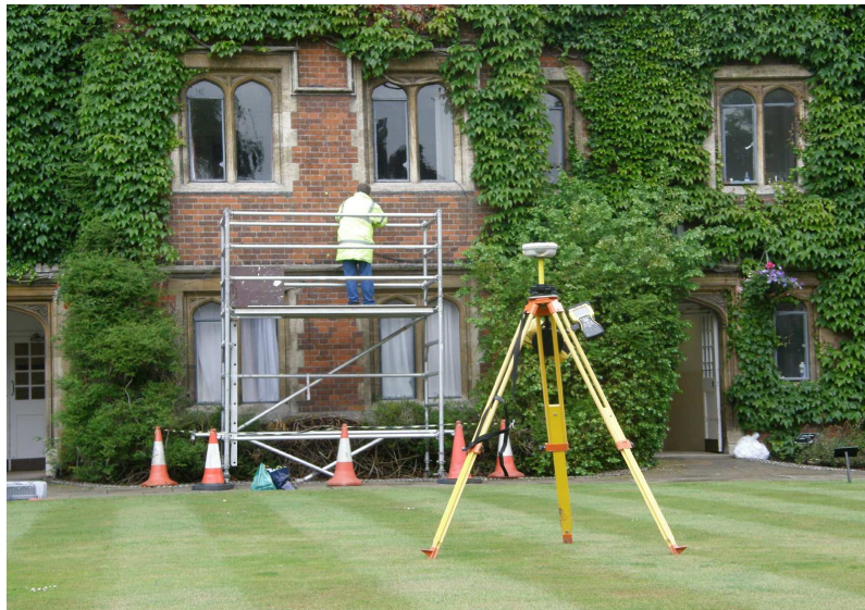
Fig. 3 — Surveying the Wall using GPS
