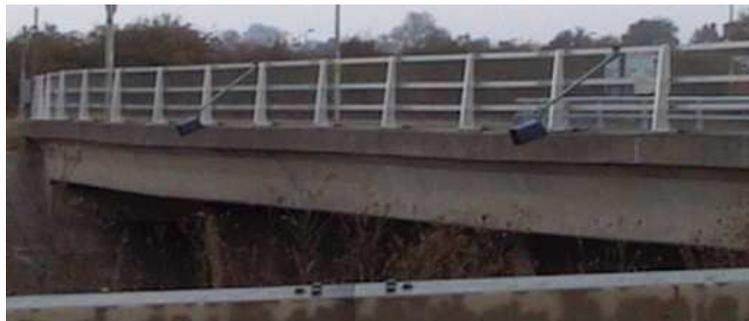
Figure 4.1: A *Trafficmaster* visual light camera installation (A14 J35, Cambridgeshire)
