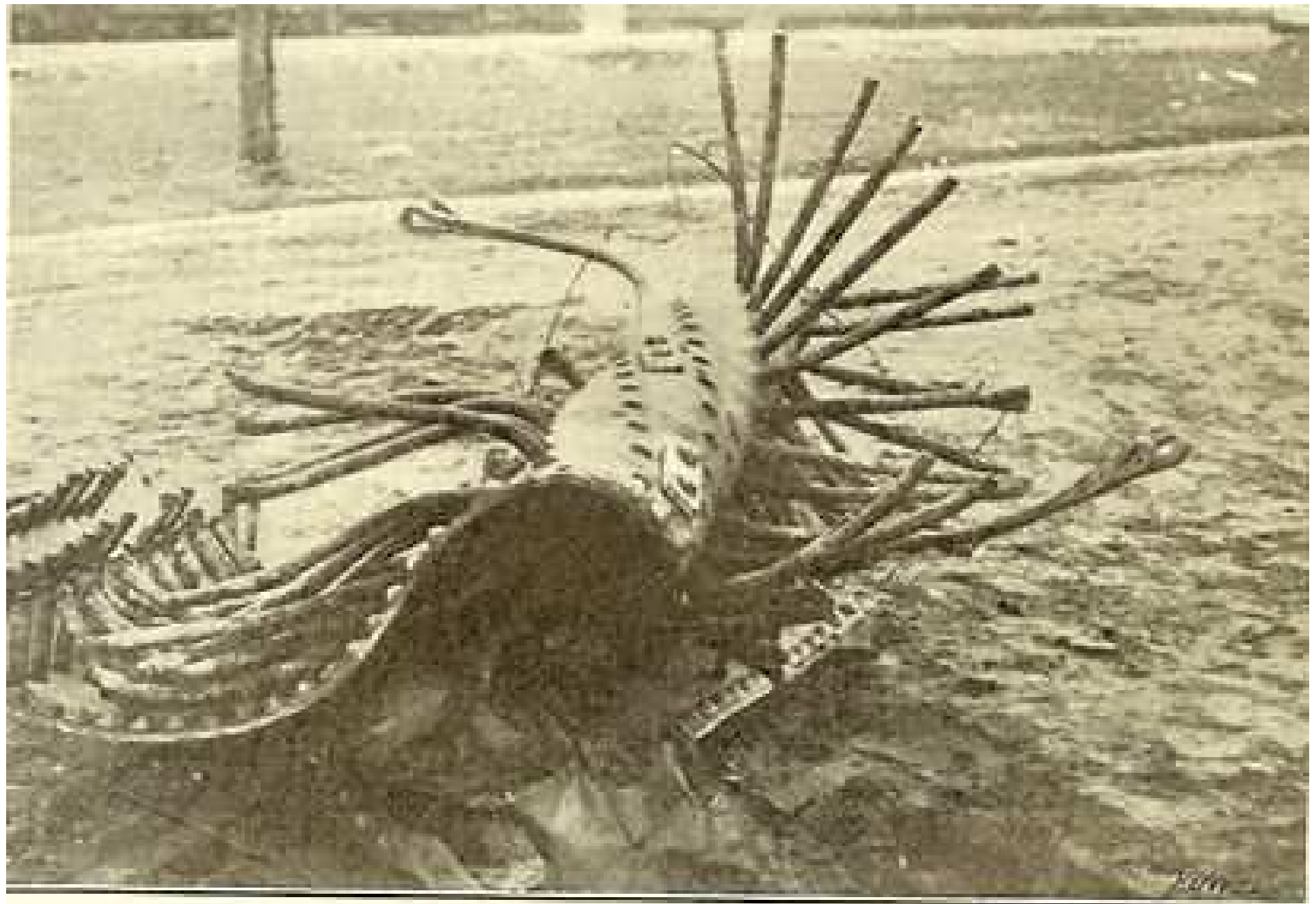
FIG. 5. AN ILLUSTRATION OF WHAT EXPLOSION DID TO STAYS AND BRACES
