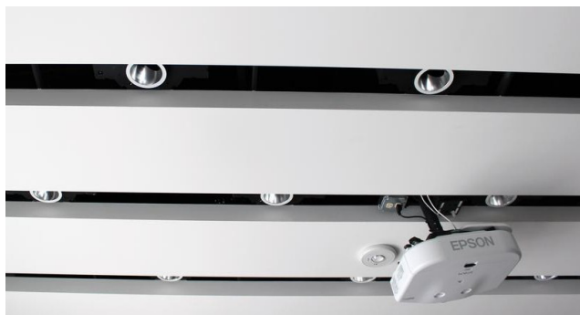
Figure 3: Recessed ceiling lights. Lights such as these are traditionally difficult to meter due to limited access to their wiring and uncertainty about the topology of the lighting circuit. Our Gecko sensors are easily and unobtrusively installed in fixtures such as these. See Figure 2(c) for a closeup view of the sensor mounting.
