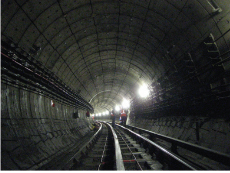
Fig. 1. Underground railway tunnel in London
