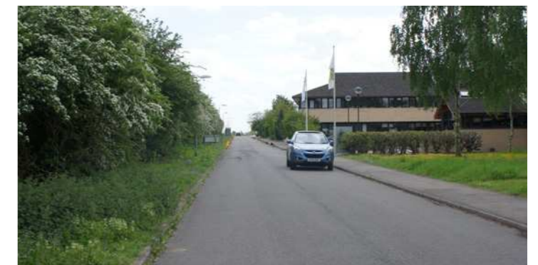
83. Western Access Road - existing photo looking south
