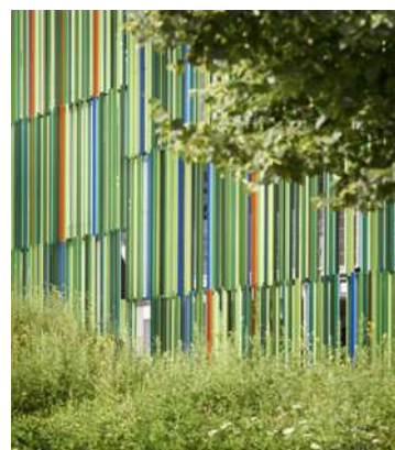
26. Parking structure in La Coruna:
