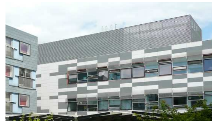
34. Rooftop Plant - screening of a large amount of rooftop plant space
