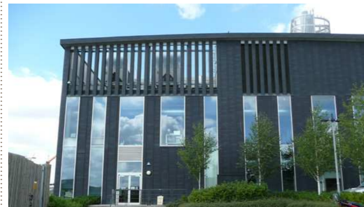
33. Rooftop Plant - medium plant integrated within the elevation of the building
