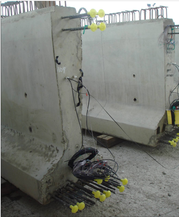
Figure 1.4: BOTDR fibres emerging from the ends of precast beams; the black fibres are for temperature compensation
