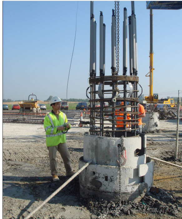
Figure 1.5: Pile cage instrumented with BOTDR fibres undergoing careful installation into its borehole
