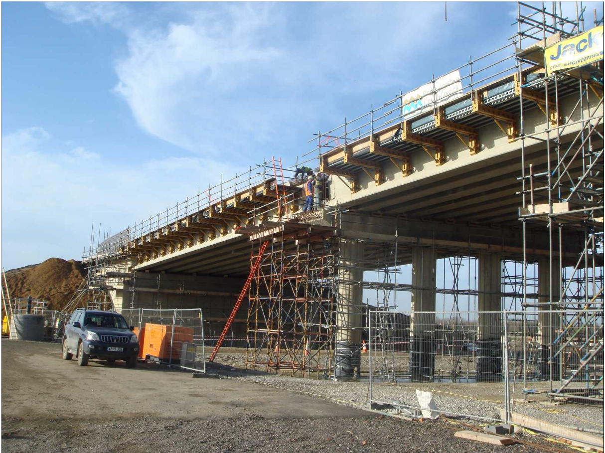
Figure 1.3: Addenbrooke's Access Road bridge during construction; strain-sensing fibres are embedded in some of the cast concrete beams visible and also in several of the piles supporting the far abutment and the near pier.
