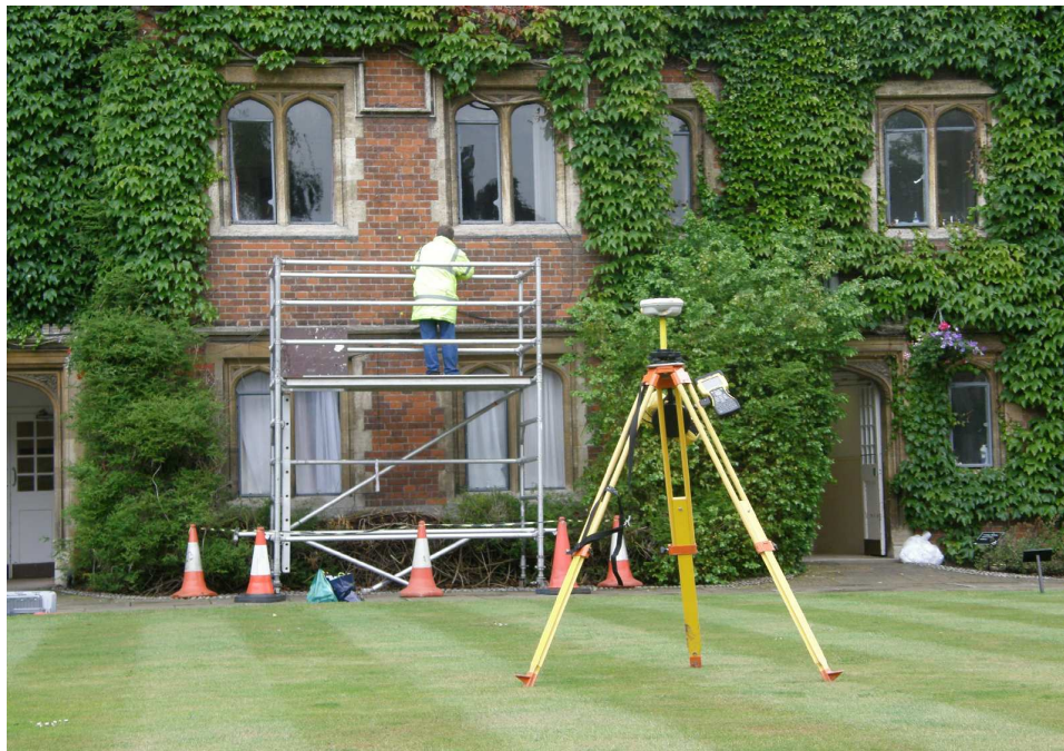
Fig. 3 — Surveying the Wall using GPS
