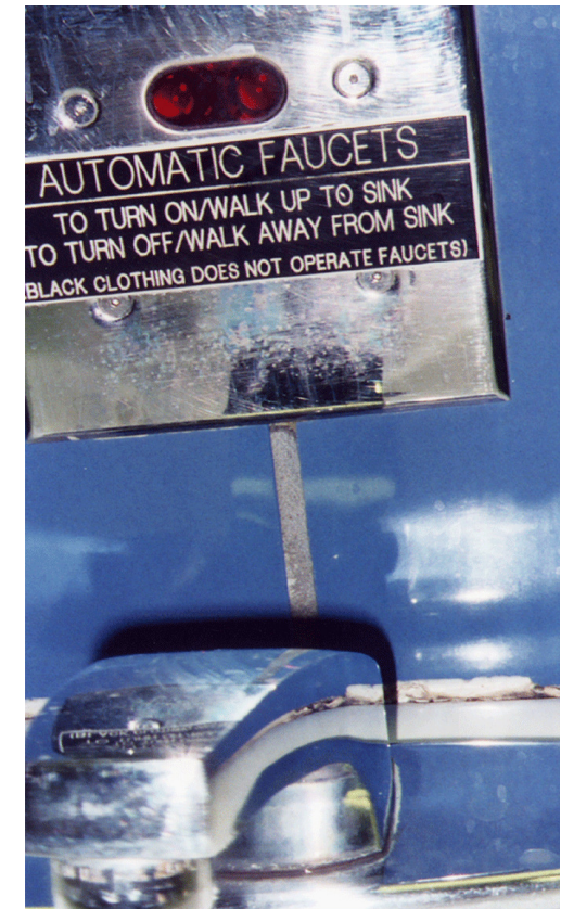
Figure 1.10 A sign in the restrooms at Cincinnati airport. Because it is not visible to the user as to what to do to turn the faucet (tap) on and off, a sign has been added to explain what is normally an everyday and well-learned activity. It does not explain, however, what to do if you are wearing black clothing
