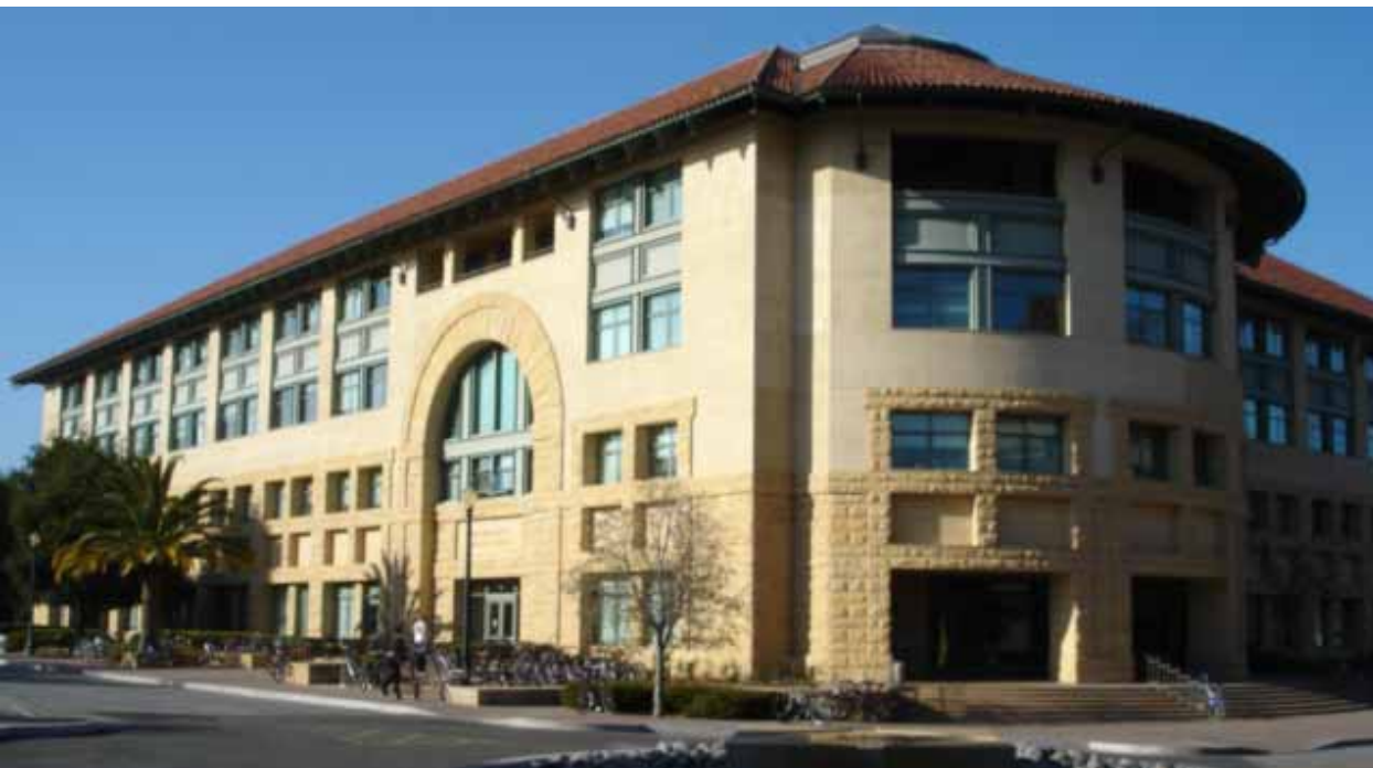
Gates Building – the rounded version (Stanford)
