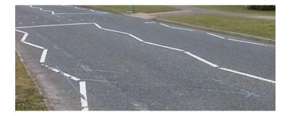
Figure 4.3: A magnetometer induction loop detector buried in a sawn groove in the tarmac and grouted with sealant
