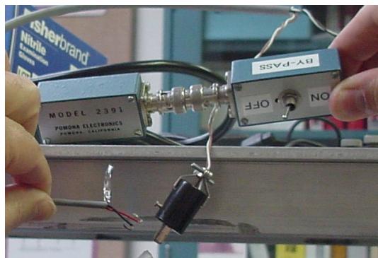
Figure 1: The interlock bypass switch showing box that was floating at 12V.
