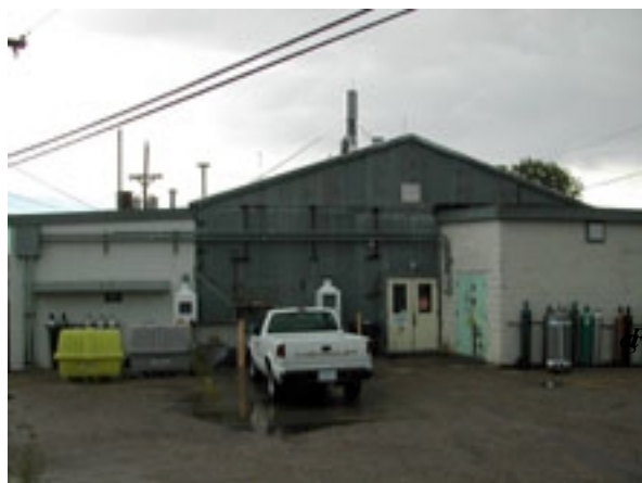
Figure 2.3. Building 41 at TA-46.
